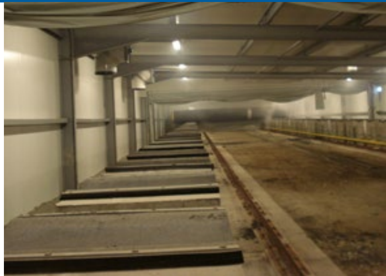
Curing steam tunnel
