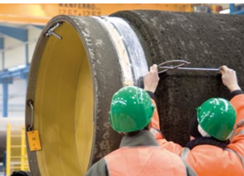
Inspection coated pipe
