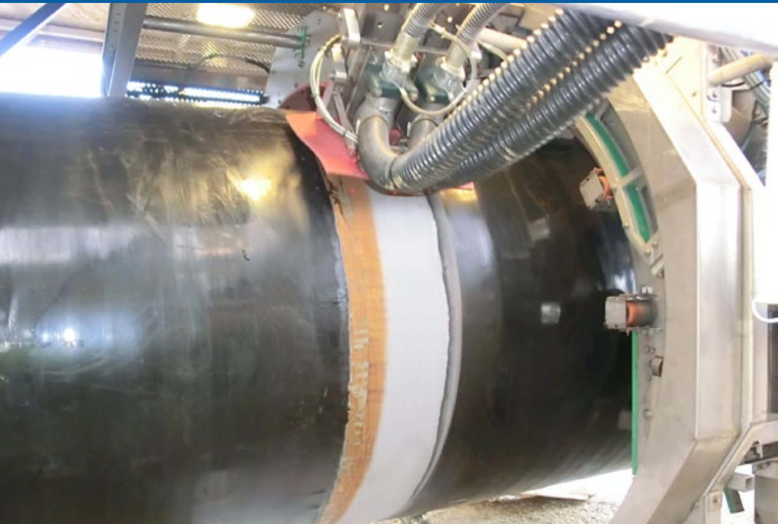
Vacuum blaster on site
